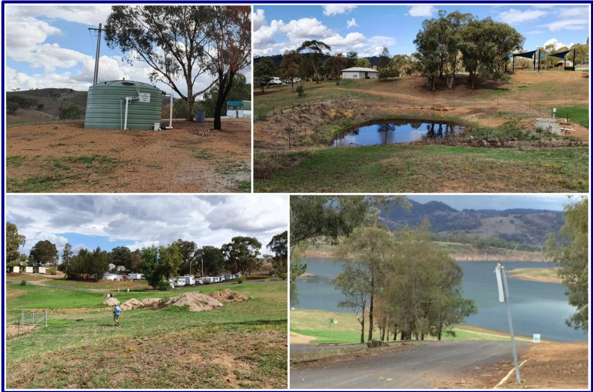
Figure 22 – Assets Encroaching on State Water Land Top LHS clockwise: Water Supply Treatment Plant Storage Tank, Dam and Sewer reticulation pond, Dual Road to boat ramp and access road to Long-term site precinct.
