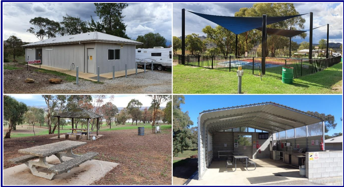
Figure 18 – Assets Holiday Park Recreation Area Top LHS clockwise: New amenities block; children’s playground; Camp Kitchen; bench seating, shade.
