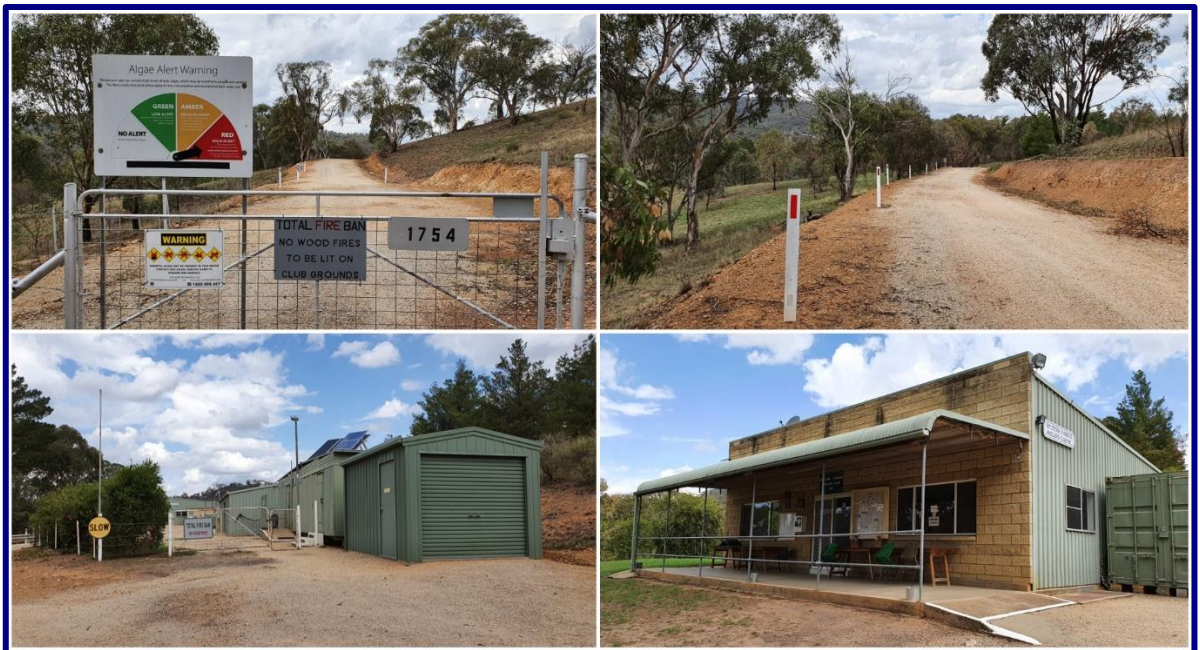
Figure 21 – Assets Anglers Club Top LHS clockwise: Entrance gate and signage; all-weather access road; Clubhouse; Amenities/ sheds. Lot 3.
