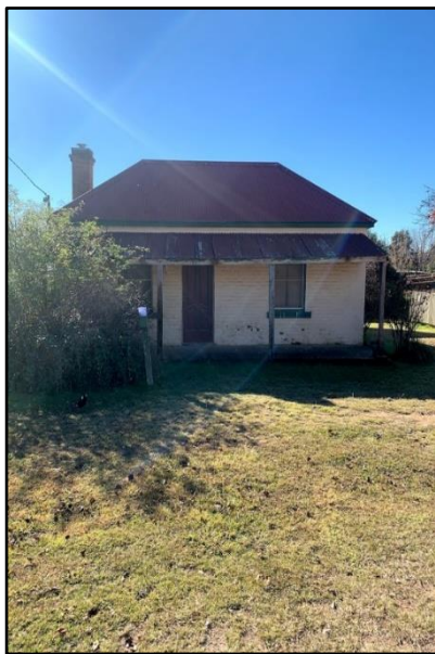
Figure 23. External view of the primary (southern) façade of heritage item I81 located at 6-8 Inglis Street, Mudgee, as viewed facing north from Inglis Street.
