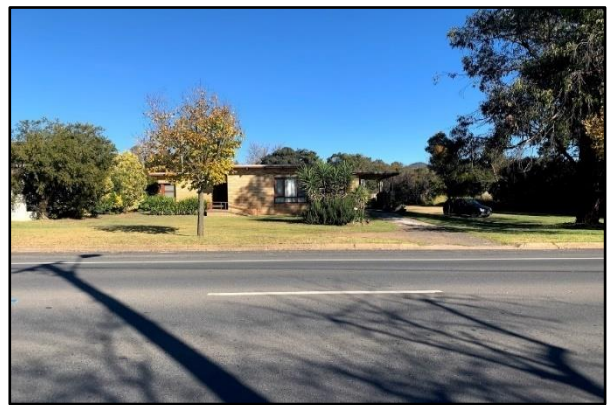
Figure 18. External view of the primary (northern) façade of the dwelling on the subject site (Post-War residence). Taken facing south from the north side of Horatio Street.
