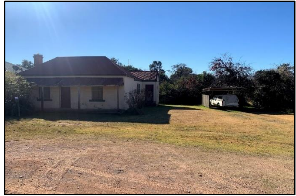
Figure 22. External view of the heritage item I81 located at the rear of the subject site, facing north from Inglis Street.
