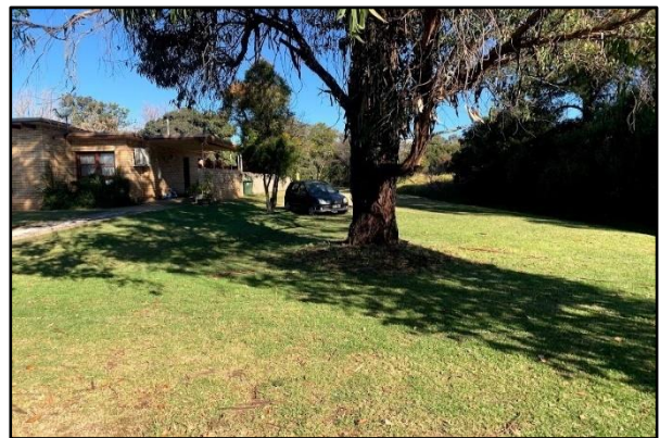
Figure 20. External view of the garden space on the eastern side of the subject residence. Taken from the south side of Horatio Street, facing south.
