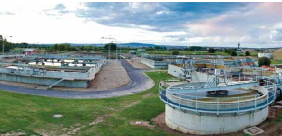
BELOW Wastewater Treatment Works, Bathurst
