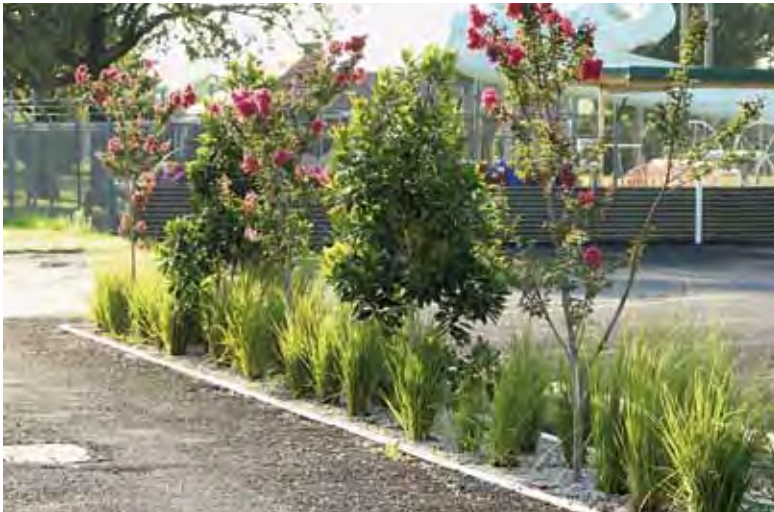
ABOVE Raingarden at Dubbo City Council's public pool (Photo C. McCulloch)
