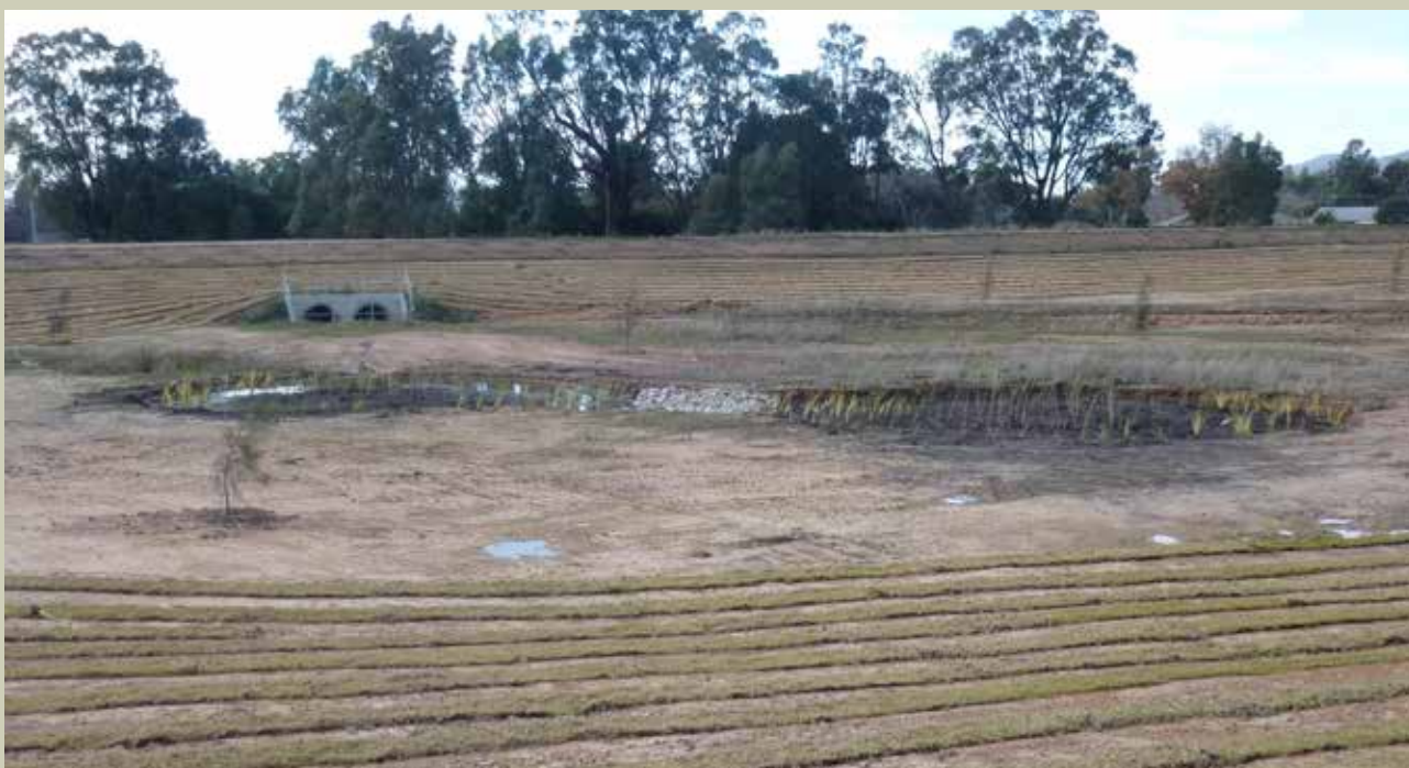
Detention basin restoration, west Mudgee.
