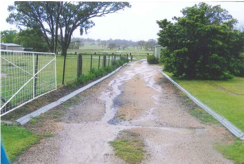
Figure 3-3 Stormwater running along the Driveway of 15 George Street
